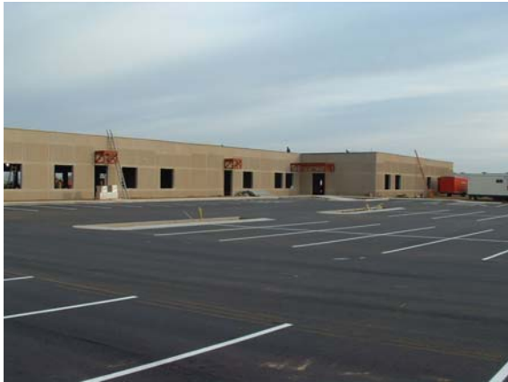
Construction of the 30,634 sq. foot Centre in progress
