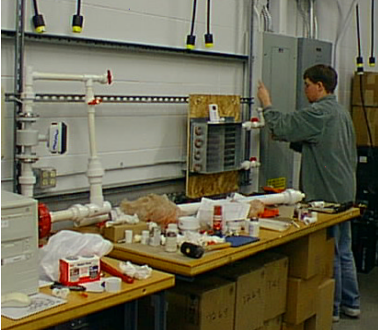
The Heating/Cooling Demo loop slowly takes shape.
