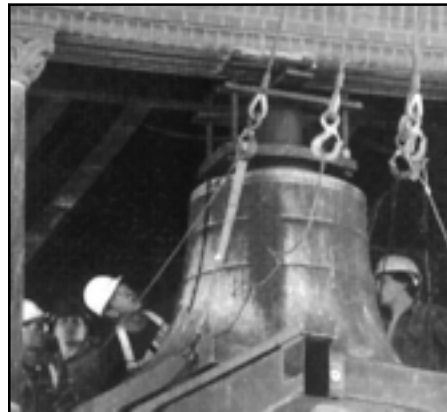
Workers remove the cracked bell from Bowman Hall.
